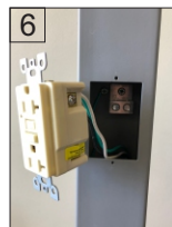
6 Install the wiring device and wire accordingly.
