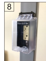
8 Finished Installation. Recommended to put silicone in all opening.
