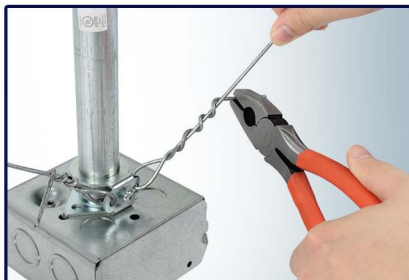
5 Mount seismic wires to surroundings and tie to holes of CLCSL
