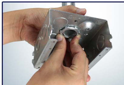
4 Secure conduit to box using locknut
