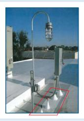
Perfect for control, fire alarm, service receptacles and power to electrical equipment installation on roofs
