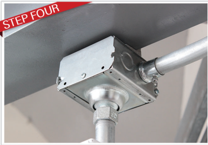
(4) Attach Side Plate with screws to finish installation
