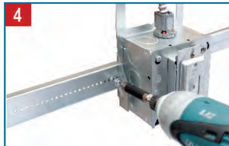
Secure the assembly to the BHA with Tek screws, setting the box in place
